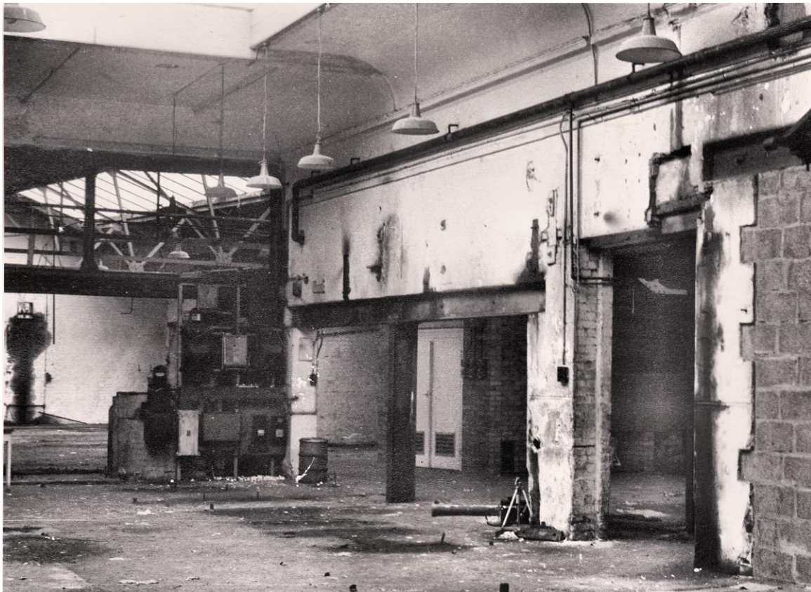
The building with all machinery removed, prior to conversion work commencing
